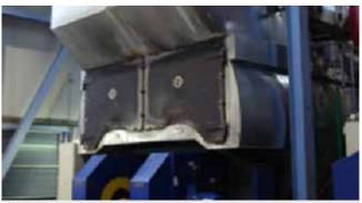
Coke oven gas firing system in Germany with SAACKE Low-NO<sub>,</sub> gas burners
